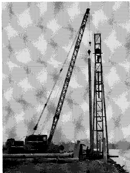
Figure 2-16 in octagonal pile-driver with 4-ton monkey.
