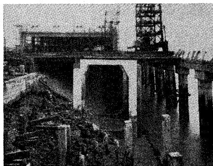
Figure 5—Looking downstream beneath the jetty head.
